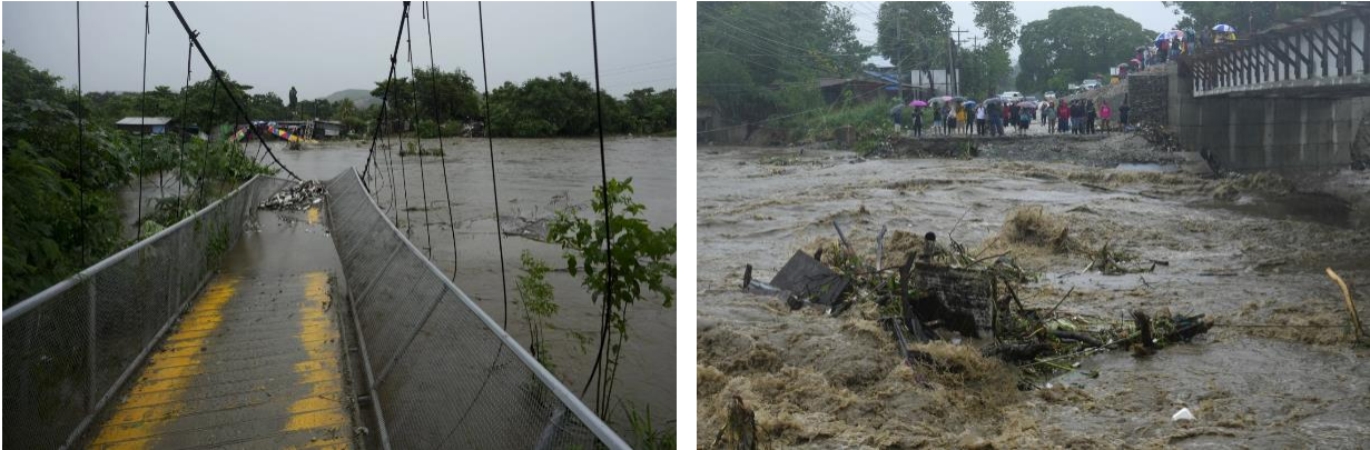
Figure 3 Pedestrian bridge collapsed due to flooding in San Pedro Sula
