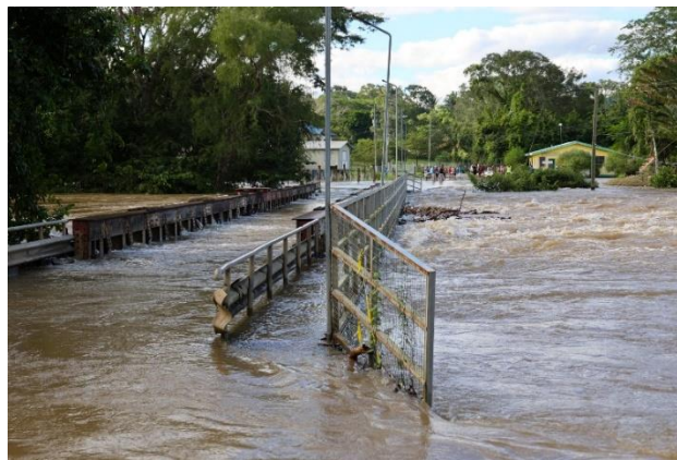
Figure 3 Flooding area and blocked road
