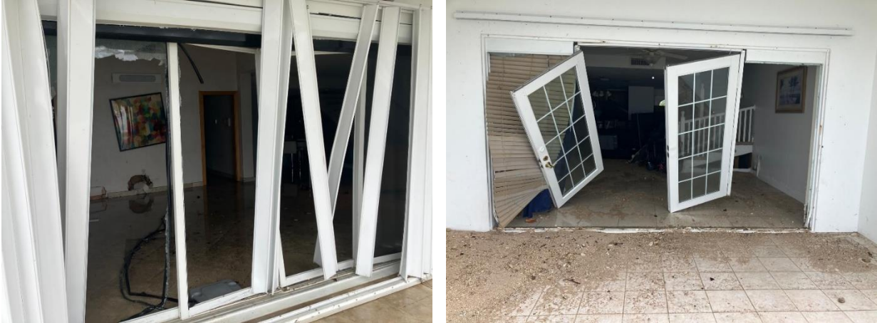
Figure 4 Shutters splintered in the storm and doors blown apart at Windsor Village. – Photo: James Whittaker
