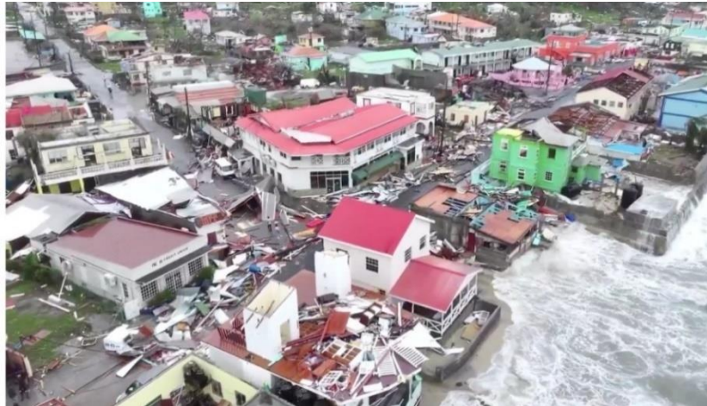
Figure 5 Rubble-strewn streets of Hillsborough, Carriacou, shows the devastation caused by Hurricane Beryl
