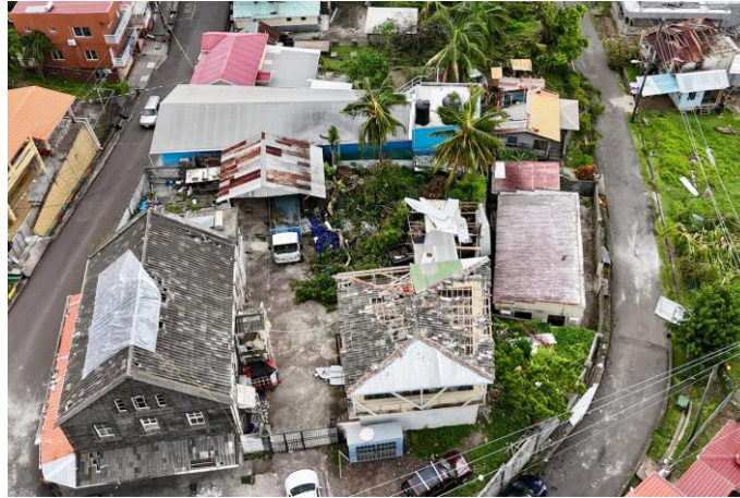
Figure 8 Buildings with damaged roofs in Grenada (Ian Hughes/Reuters).
