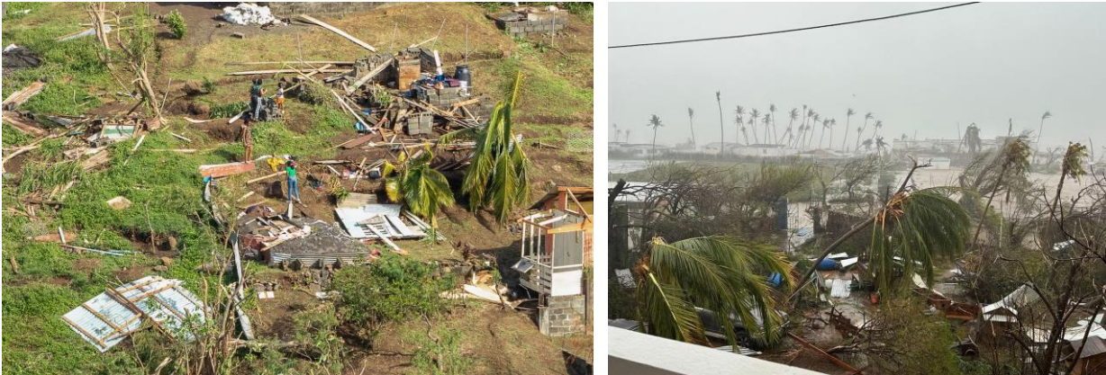
Figure 7 Damaged dwellings in St. Vincent and the Grenadines. (Lucanus Ollivierre/AP, left - Ralph Gonsalves/Reuters, right)
