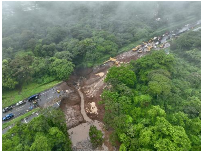
Repair actions on the Palín-Escuintla highway / Foto: CIV
