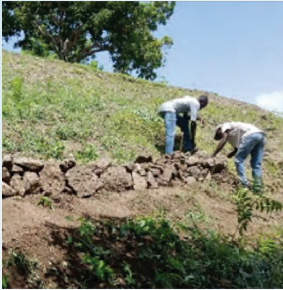
Creating a stone and earthbag wall to prevent erosion
